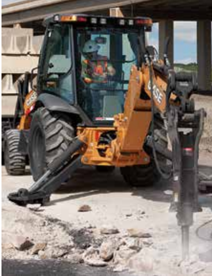
Optimized hose routing for demolition work
